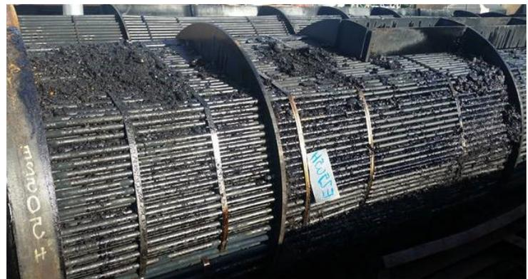
Preheater train heat exchanger E-2505H decontaminated (0% LEL, 0% H<sub>2</sub>S, 0% benzene) using Vapor-Phase method in 11 hours without viscosity wash with LCO and Rezyd-HP Z71.\*
