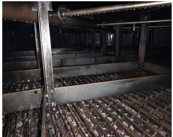
◆ VDU PACKED BED SECTIONS CONTAINED NO SCALE OR PYROPHORICS AFTER ZYMEFLOW'S PROCESS
